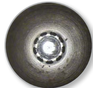
Inspection of injection nozzles
