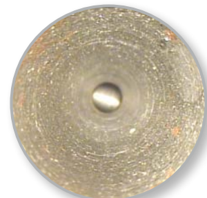
Deposits in pipe
