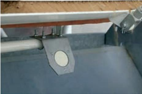
Sensor installed in material chute under silo outlet
