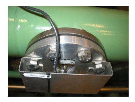
Determination of water content in oil or diesel e.g. in oil separator or central lubrication plants
