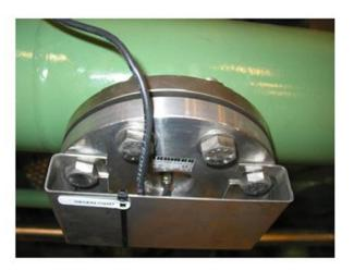
Determination of water content in oil or diesel e.g. in oil separator or central lubrication plants
